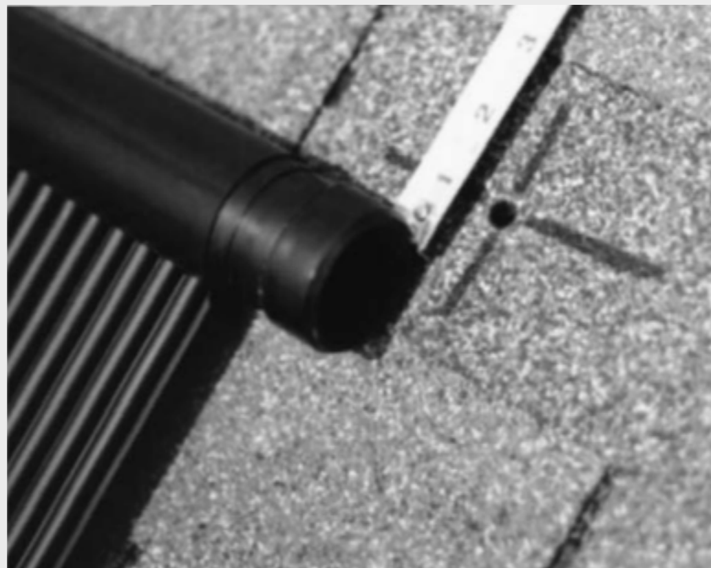
FIGURE 3 Outlet Header Bracket Location
