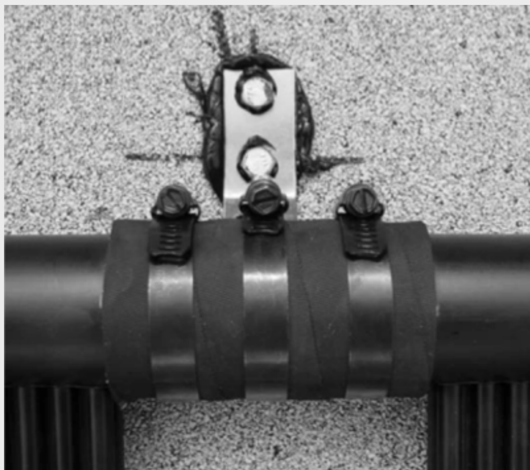
FIGURE 5 Installed Outlet Header Bracket with Hose
