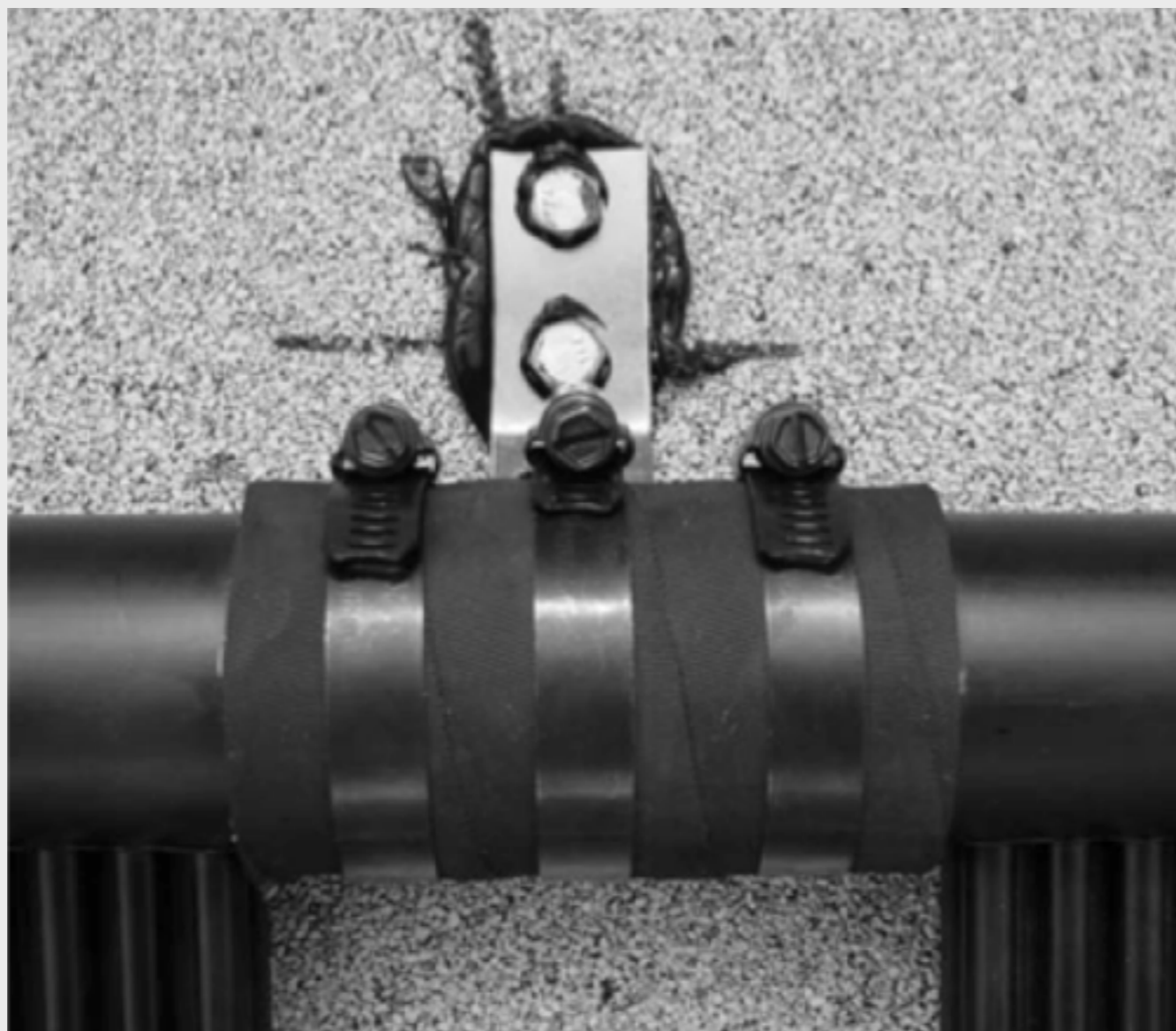
FIGURE 5 Installed Outlet Header Bracket with Hose
