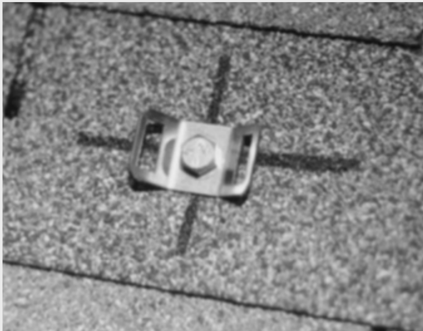
FIGURE 6 Hold-Down Strap Bracket
